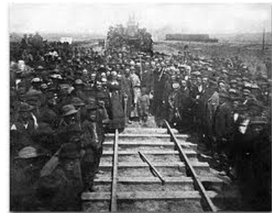
The Last Rail is Laid
