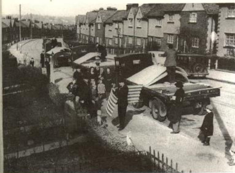
SOURCE 1 A photograph taken in February 1939. 'Anderson' bomb shelters are being delivered in London. The shelters were sunk into the ground in people's back gardens
